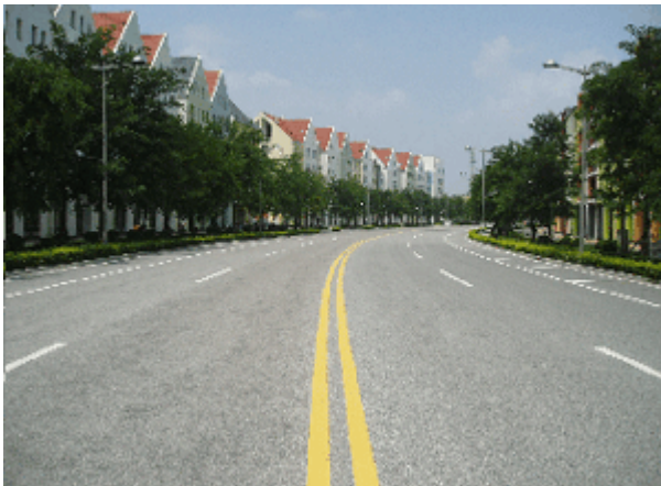
Fig. 4 : Excessively broad, curved street in the centre of the 'European' city Anting.
