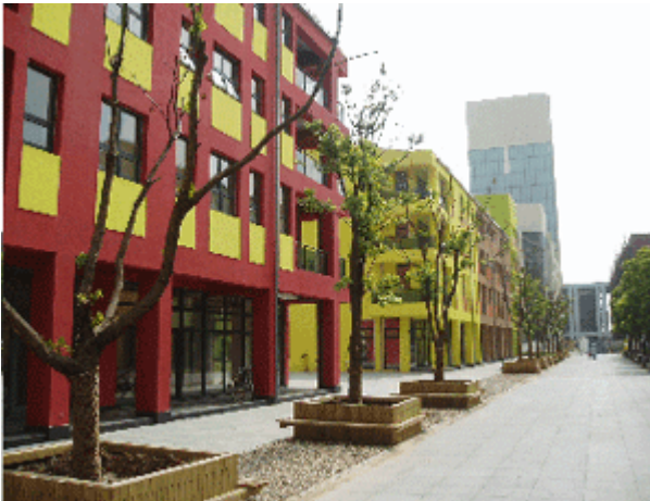
Fig. 3 : Residential buildings with commercial ground floor use.
