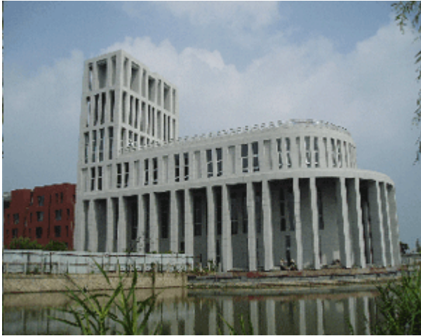
Fig. 9 : Anting Church (under construction).
